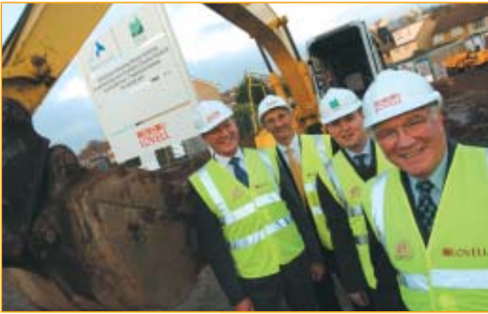
Building work for our first new homes in Tile Hill has begun
