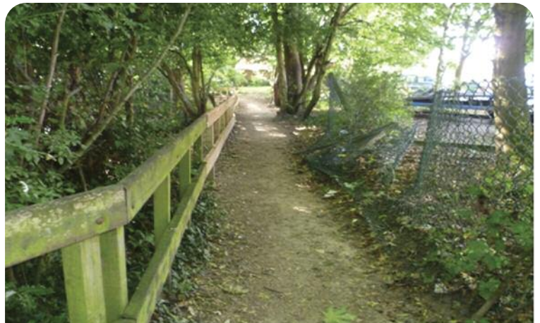
Fencing along the Sowe Valley, which will be renewed as part of the scheme
