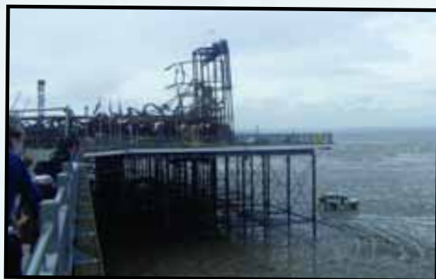
• Weston's fire damaged pier
